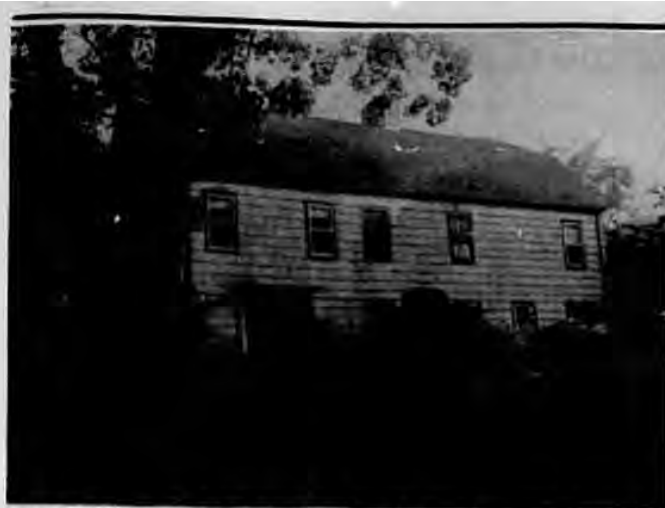
THE PRATT HOUSE on 30 Valley Road in Council, may solve some of the town's Watchung, recently acquired by the Borough recreational needs.
